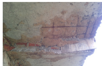
Clear visible of MS Rod at the ceiling of the vending Zone
